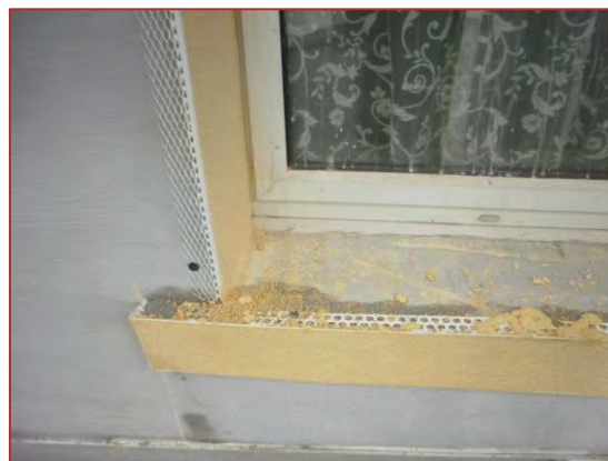
Figure 22: Window sill and reveal after receiving the finishing coat of the render system
