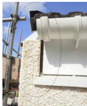
Figure 2: Example of a poorly planned and executed junction detail
