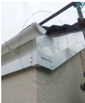
Figure 1: Example of a well planned and executed junction detail
