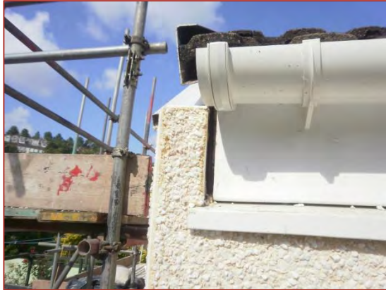
Figure 29: Eaves and verge junction at a gable wall
