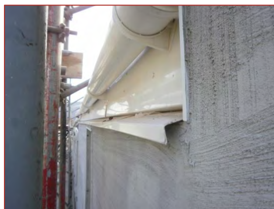
Figure 20: Retrofitted EWI detail at an external wall to eaves junction where two terraced dwellings are at different levels
