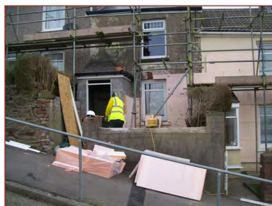
Figure 10: Early stages of the retrofitted EWI being installed at ground floor level
