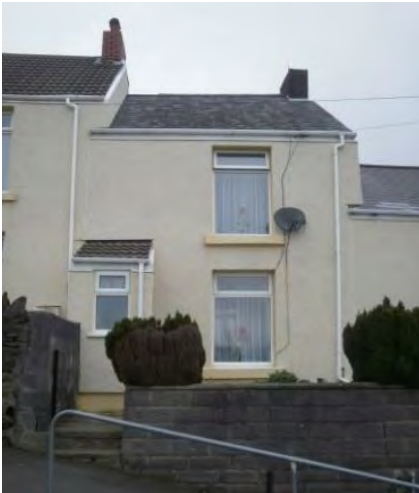
Figure 16: Photograph of a case study dwelling after EWI was installed (Hopper, 2012)
