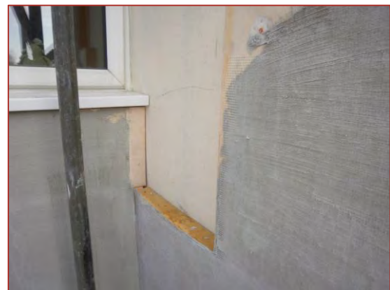
Figure 18: Retrofitted EWI receiving base coat of rendering system below PVC window sill at external wall to window junction (same window as shown in Figure 12)
