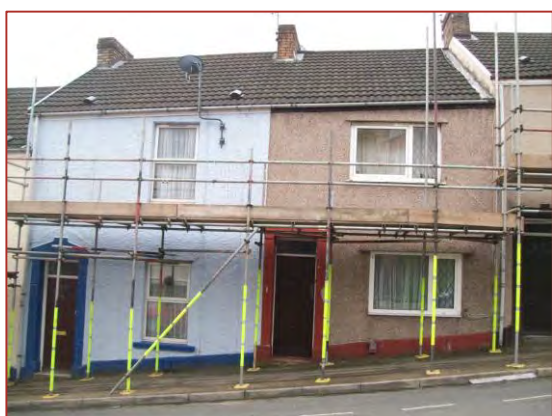
Figure 9: Two dwellings being prepared for the retrofitted EWI installations
