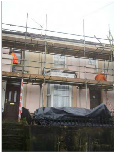
Figure 11: Early stages of the retrofitted EWI being installed at first floor level
