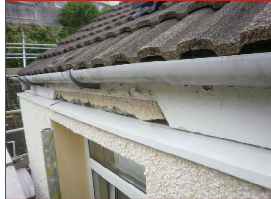
Figure 30: EWI installed above window
