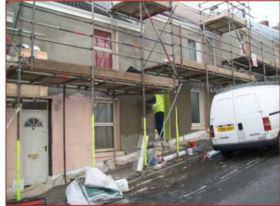
Figure 14: Retrofitted EWI receiving a base coat of the rendering system
