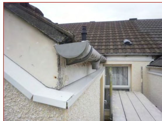
Figure 26: Capping profile junction between the eaves and verge
