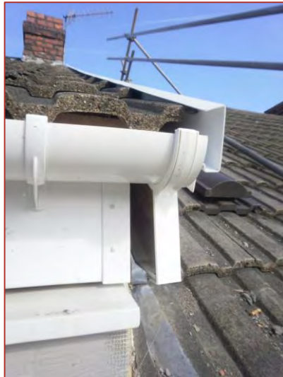
Figure 23: Eaves and verge junction between two dwellings
