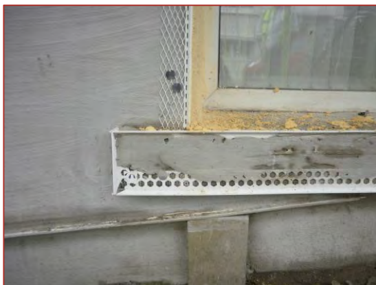
Figure 17: Ground floor stone window sill after receiving retrofitted EWI and base coat of rendering system
