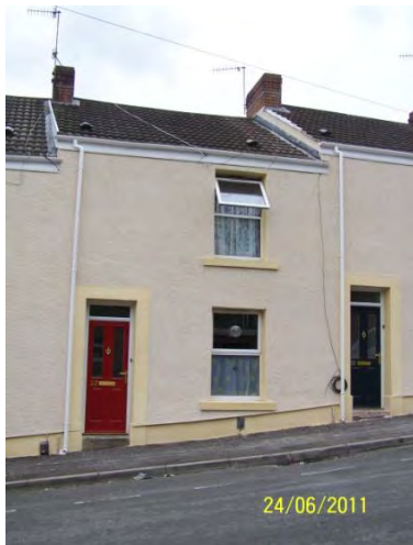
Figure 8: Photograph of Case study A after installation of EWI
