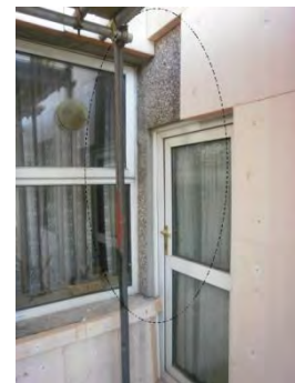
Figure 3: Example of lack of a preliminary survey and appropriate technical detail
