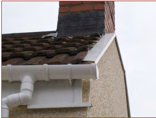
Figure 31: Verge and eaves junction with downpipe connection to the gutter
