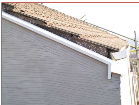
Figure 19: Retrofitted EWI detail at a gable wall and eaves junction
