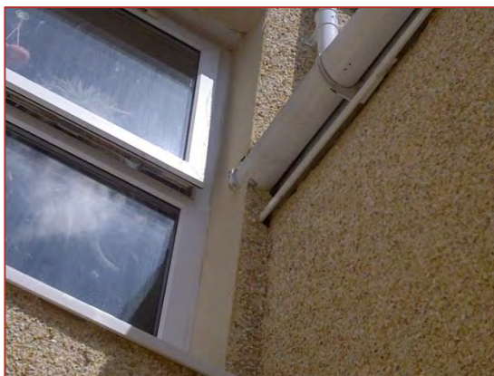
Figure 25: Existing gutter embedded into the EWI
