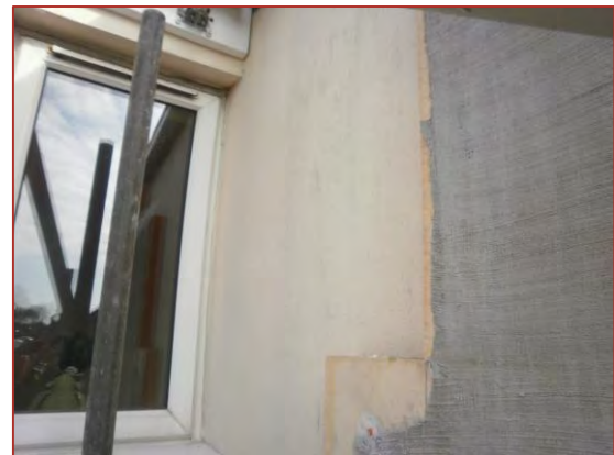
Figure 16: Retrofitted EWI receiving the base coat of the rendering system at an external wall to window junction
