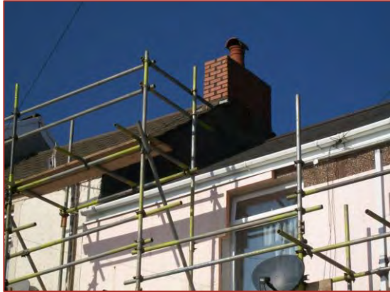
Figure 13: Retrofitted EWI being installed at the eaves of a dwelling
