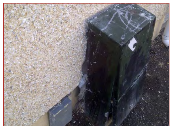
Figure 34: Telecommunications junction box located in front of an external wall
