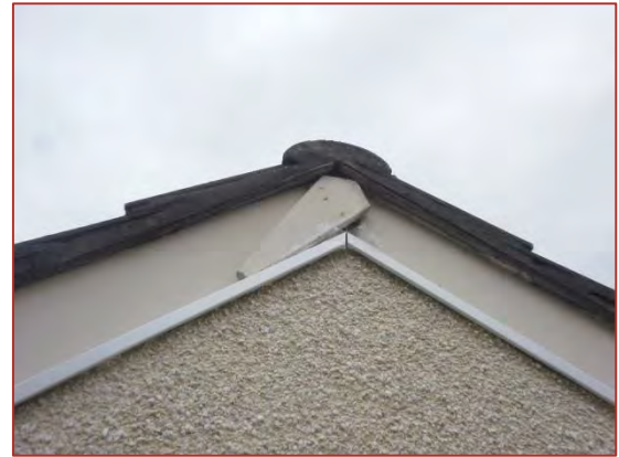
Figure 32: Verge junction at the ridge of the roof on a gable wall
