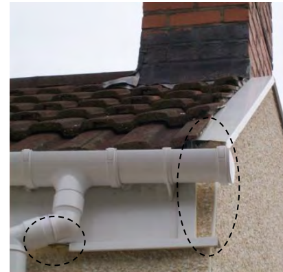
Figure 3: Example of poor detailing and execution resulting from an inadequate preliminary survey
