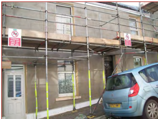
Figure 15: Retrofitted EWI after receiving base coat of rendering system
