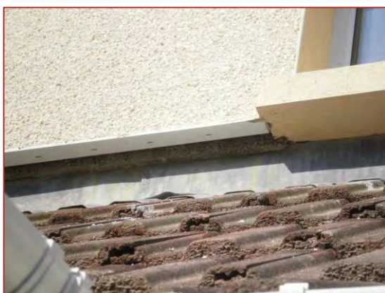
Figure 33: Drip bead detail at a single storey roof abutment junction with an external wall
